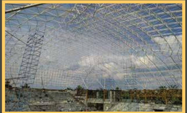
Metal Space Frame is a prefabricated three dimensional space frame system. There will not be a need for any additional work at the site including paint touch up. It is being packed in a special way to protect the powder coated components from scratches during handling at site.
