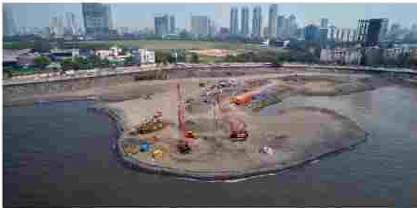
Figure 2: Drilling of stone column with rig (refill)
