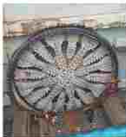
Breakthrough of Pioneer (one of Guangzhou Haizhu Bay Tunnel)
