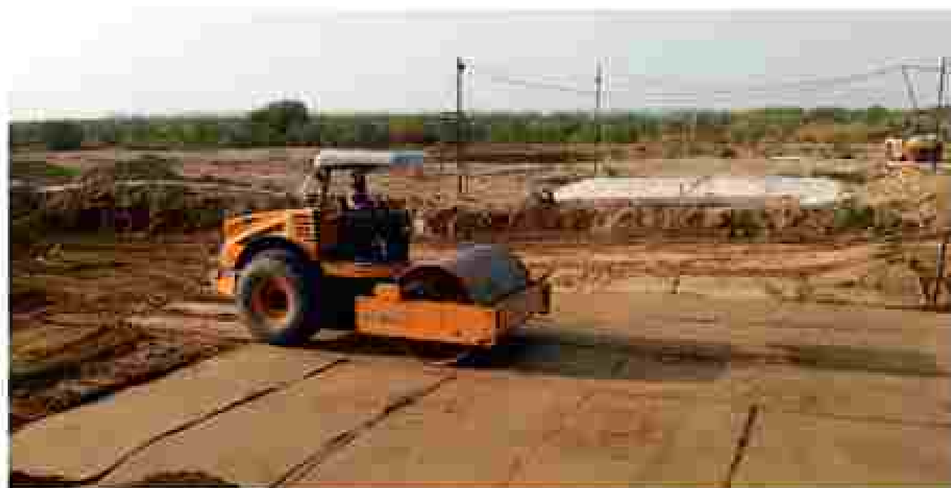
Figure 1: Soil-Cement Stabilization Ground Improvement Method
