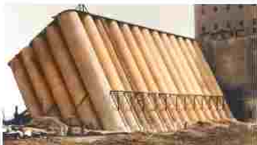
Figure 3: Collapse of Transcona Grain Elevator, Canada. Photo Source: enr.com
