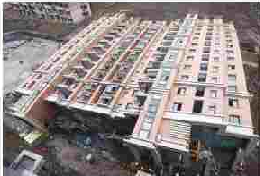
Figure 6: Tilting of a concrete 13-story building in China. (Source: Failure, Cause, Building collapse in Shanghai" 20 Apr 2008, www.enr.construction.com/resources/special/ )
