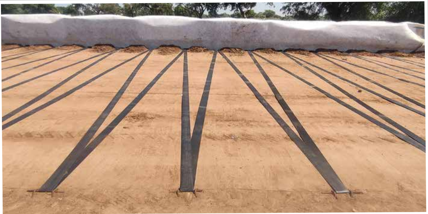
Fig 4. Typical cross section of laying of ATSTRIP
