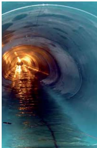
values) reduces insulation costs and heat loss. Another major benefit of GRE pipes is the fact that, once they are installed, they are almost maintenance-free. GRE pipes are well suited for environments where corrosion resistance is required at a reasonable price. Main uses include petrochemical process lines, oil and gas systems, fire-fighting systems, offshore and onshore systems, and ship and marine applications. GRE pipes are available in diameters ranging from DN 25 to DN 1000.
